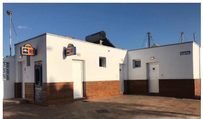
Toilet block and ATM, Pasito Blanco Agustin Martin
