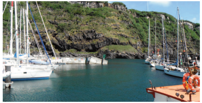
Looking across the Marina das Lajes towards the damaged northwest mole Mike Downing
