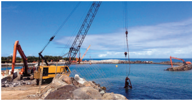
The long, curved breakwater at Cais da Barra starting to take shape in July 2018 Jornal da Ilha Graciosa
