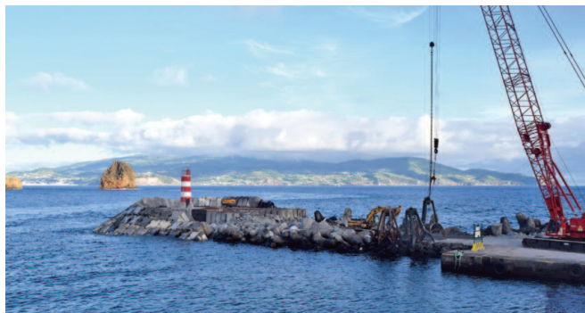
Work taking place to extend Madalena's north breakwater in June 2018. The light structure has already been moved some distance to the west, presumably to its final position. The Ilhéus da Madalena are on the left with Faial beyond Anne Hammick
