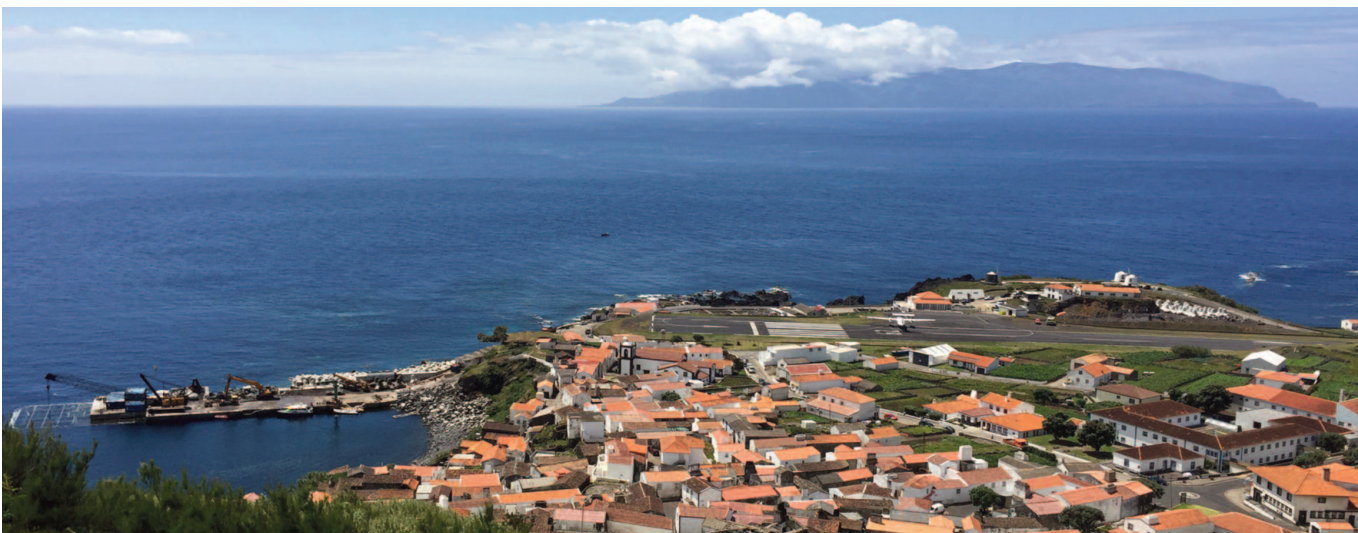
The extension to the short breakwater at Corvo's Vila Nova do Corvo taking shape in June 2018, with Flores on the skyline Mike Downing
