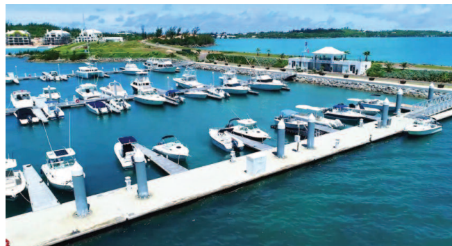
Looking NNW over the new Caroline Bay Marina in Little Sound, Bermuda Caroline Bay Marina
